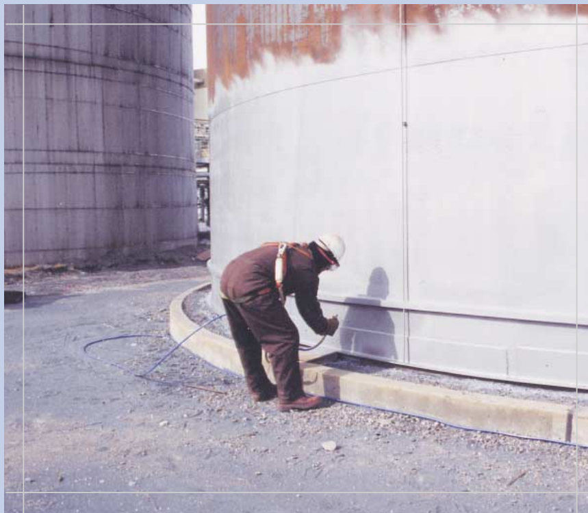
Photo: Darren Greer Sandblasting
